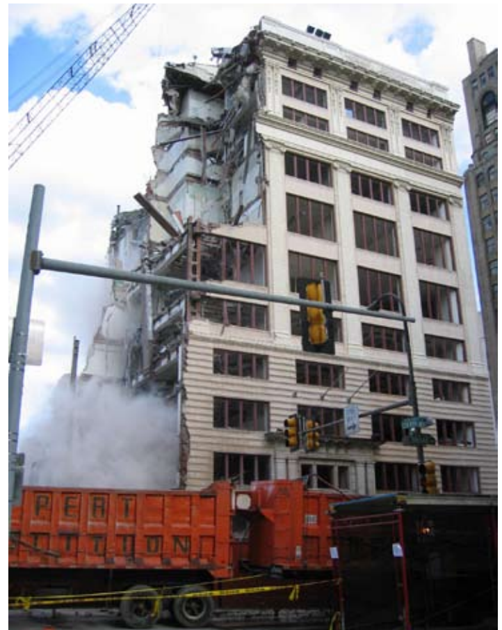
Demolition of Odd Fellows Temple, Broad & Cherry Streets, 2008, Photograph by Michael J. Seneca.
